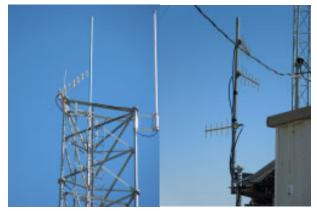
systems in use for VHF, UHF, and control along with three sixelement Yagi's for linking.
