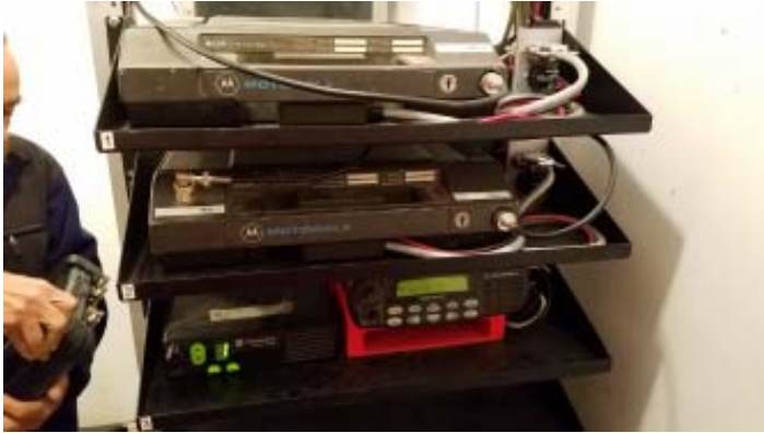
Motorola Micor radios used for the control and VHF repeater with Motorola CDM radios below for the UHF repeater.
