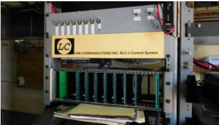
RLC-3 Link Communications controller with power switch panel above and radio card cage below.
