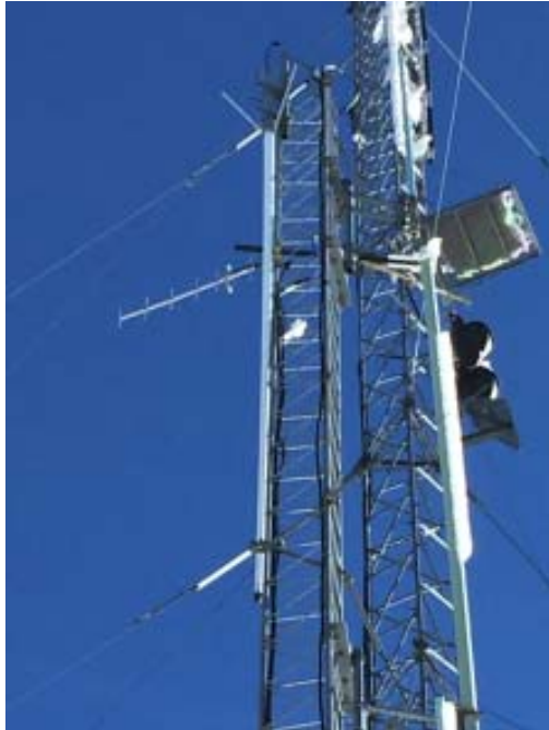
Inverted 146.980 antenna - December 30, 2015.
