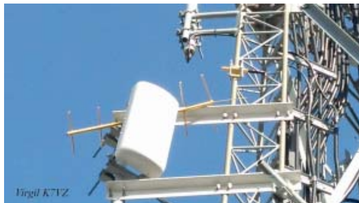
Broken Mt. Ord link antenna. February 18, 2013.
