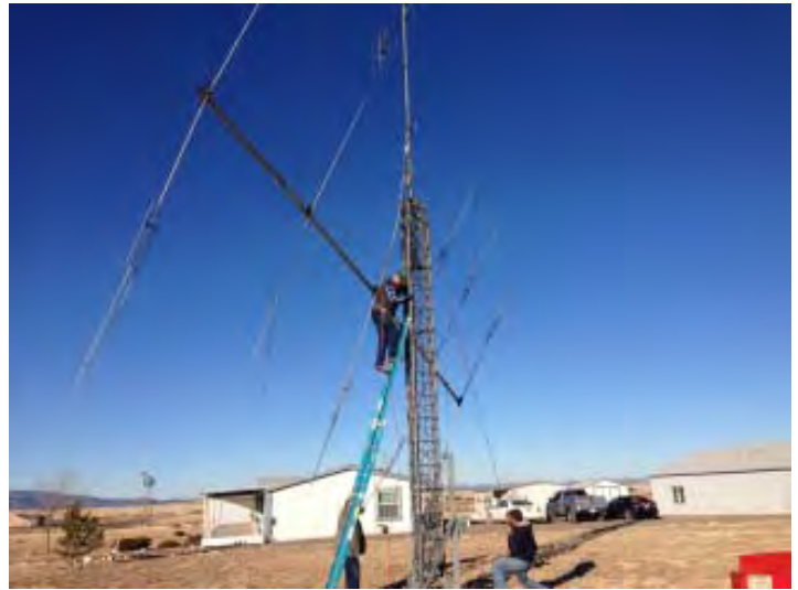
The Beam Coming Down Neil K7SEN on Tower, Bud N7CW on Rope, and Bob KJ7SJ Behind Ladder
