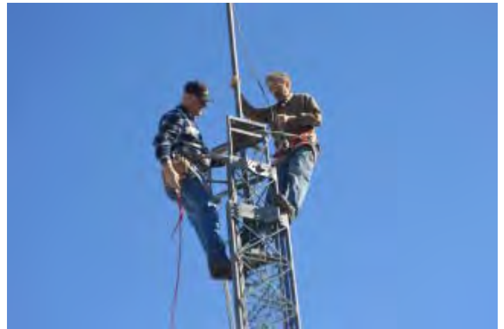
Getting Ready for the Beam Neil K7SEN and Bud N7CW on Tower
