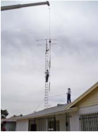
Gary, K7GH steadies the tower while the crane and Yogi, KD7ZXU do their work
