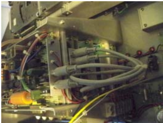
Close Up of Transmitter Showing Boards
