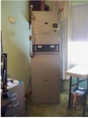
Front of Repeater/Power Supply Rack
